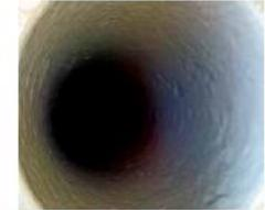
THE PHOTOS ABOVE, FROM LEFT, SHOW THE SAME WATER PIPE BEFORE CLEANING, AFTER A TOMAHAWK CLEANING AND AFTER THE TOMAHAWK BARRIER COATING. THE IMAGES ARE FROM THE JULY 2015 WATERLOO DEMO. CREWS WERE ABLE TO LINE 50 M OF PIPE IN 10 MINUTES.
