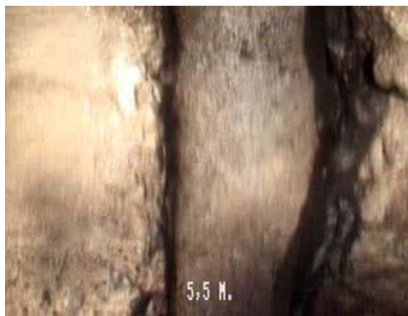
Figure 69 – (Photo 1) Trou au joint
