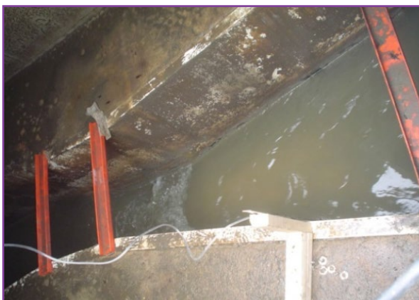
Figure 49: Canal Parshall
