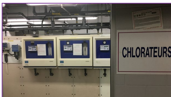
Figure 25: Chlorateurs
