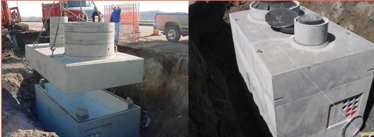
Figure 2.5: Chambre de raccordement (PA)
