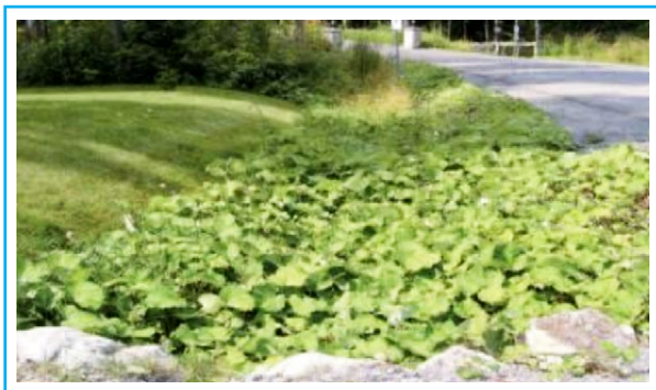
Figure 10.5: Fossé engazonné (Prévost, QC, Canada)
