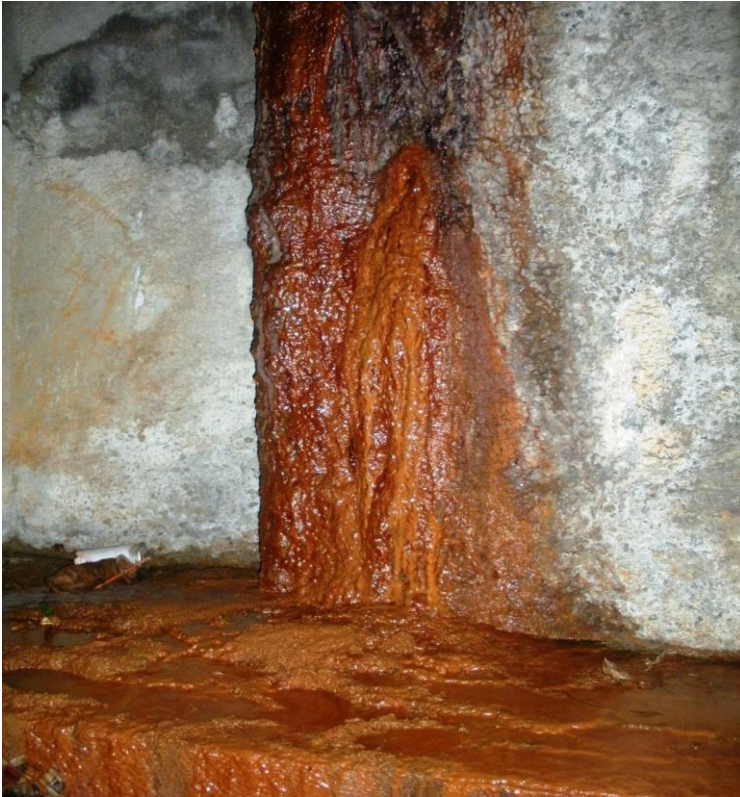
Tunnel Leakage
