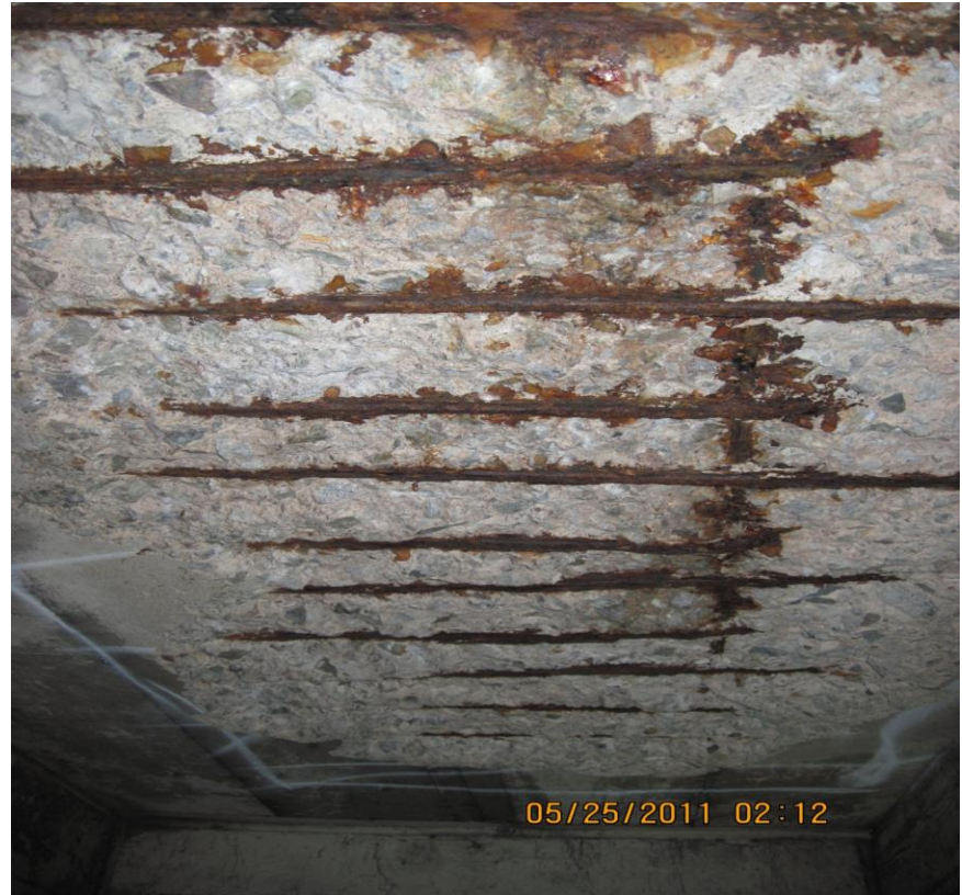
Concrete cover Spalling and Reinforcement Corrosion
