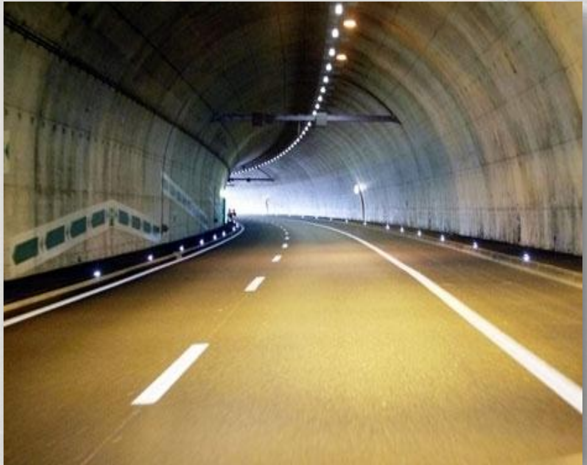
tunnel de Sévaz, 2003
