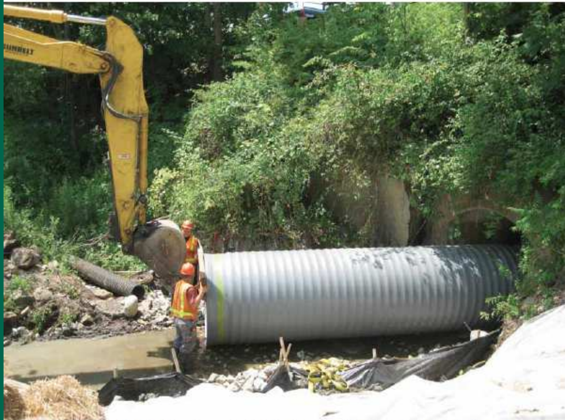
A 20-foot section of SaniFite® HP pipe being nudged into the culvert. It took the crew just hours to slipline the entire 200 feet of the culvert.
