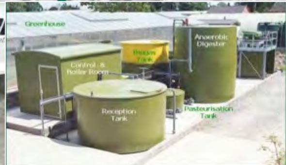
Biodigester facility : transformation of waste into energy
