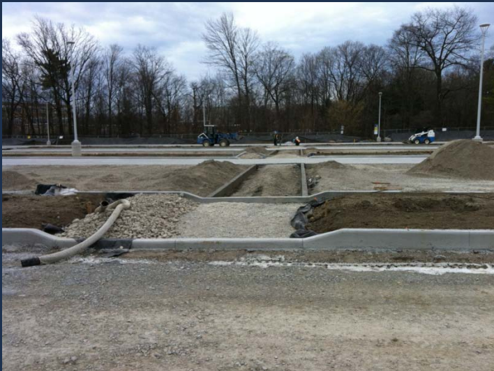
Biofilter inlet and permeable paver installation
