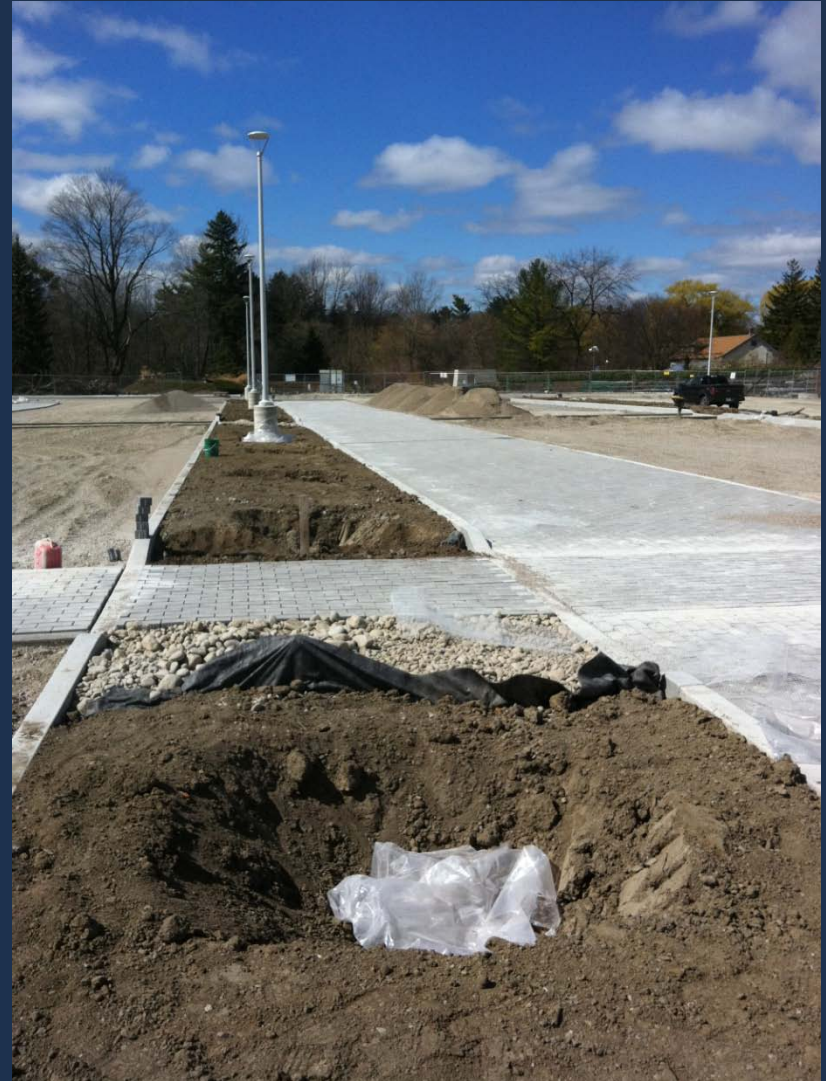
Biofilter installation
