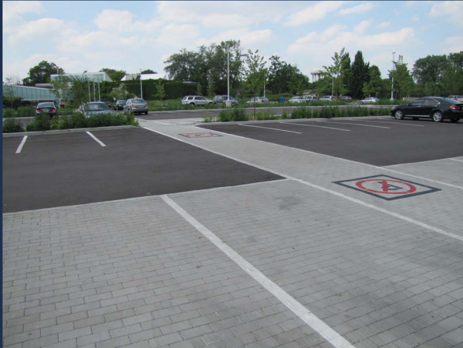
Permeable pavement parking pads and walkways
