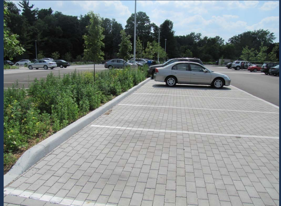
Permeable pavement and biofilter
