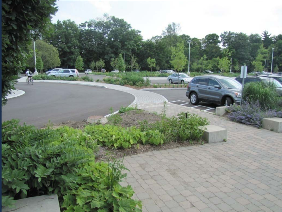
Permeable pavement at entrance roundabout
