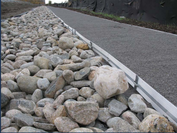
Granular Fitness Path and Drainage Swale
