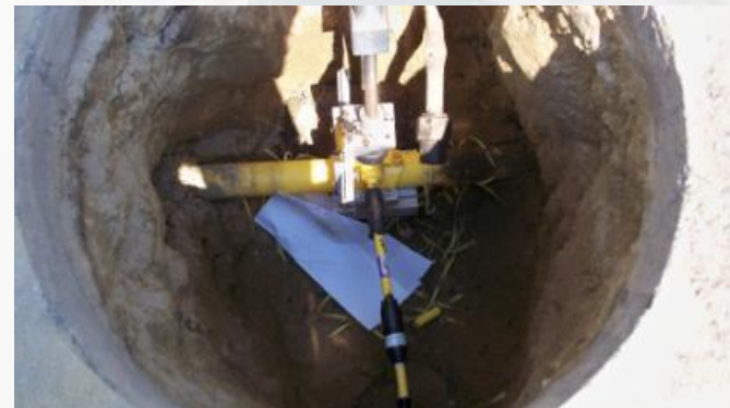
Completed service transfer
