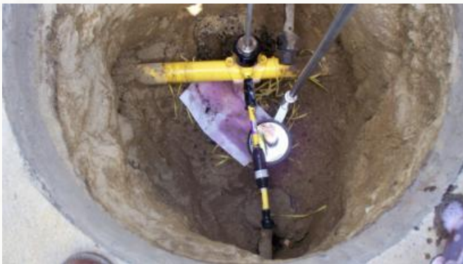
Soap test new service connections
