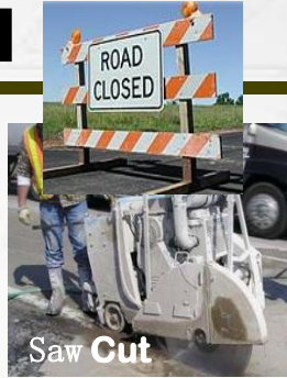
Excavate Pavement
