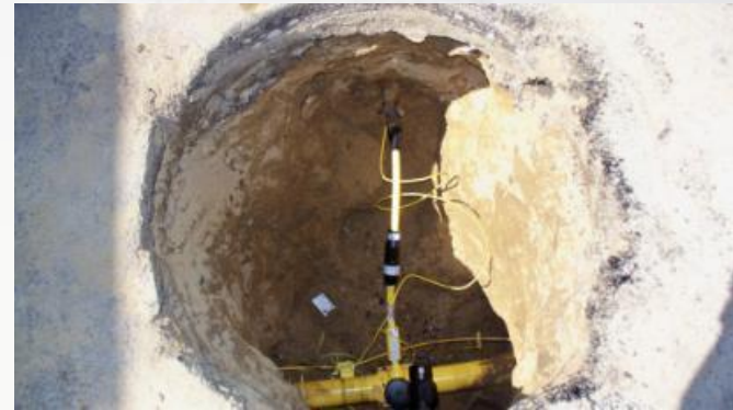
Connect 1/2" tube to service tee
