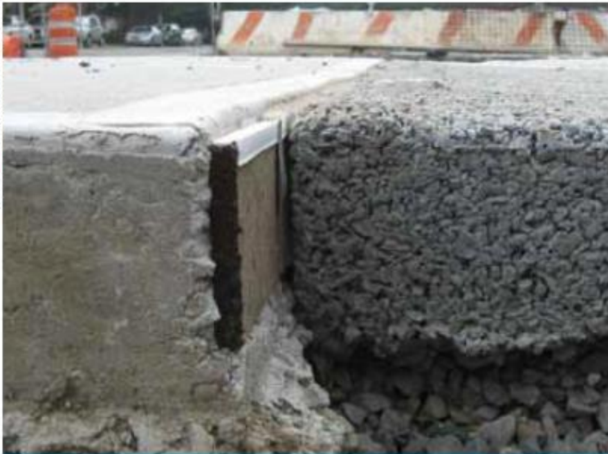
Porous concrete sidewalk Paerdegat Basin, CSO Detention Facility, Brooklyn, New York.
