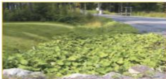
Figure 7.5: Fossé engazonné (Prévost, QC, Canada)
